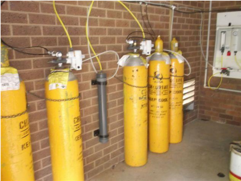
Figure 2 – Chlorine Storage Room
