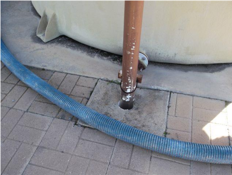
Figure 4 – Alum dosing overflow arrangements to sludge lagoon
