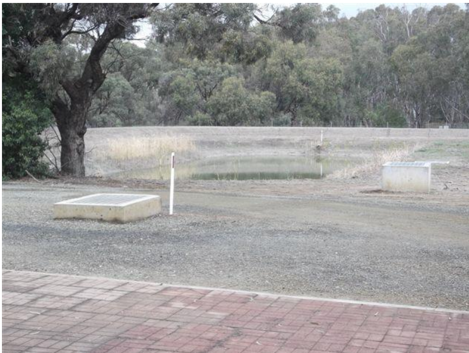
Figure 7 – Sludge Ponds showing containment bunding in the distance.
