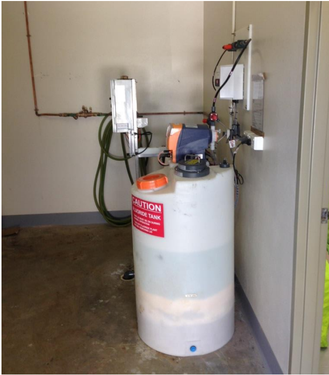
Figure 6 – Fluoride Dosing Containment Tank
